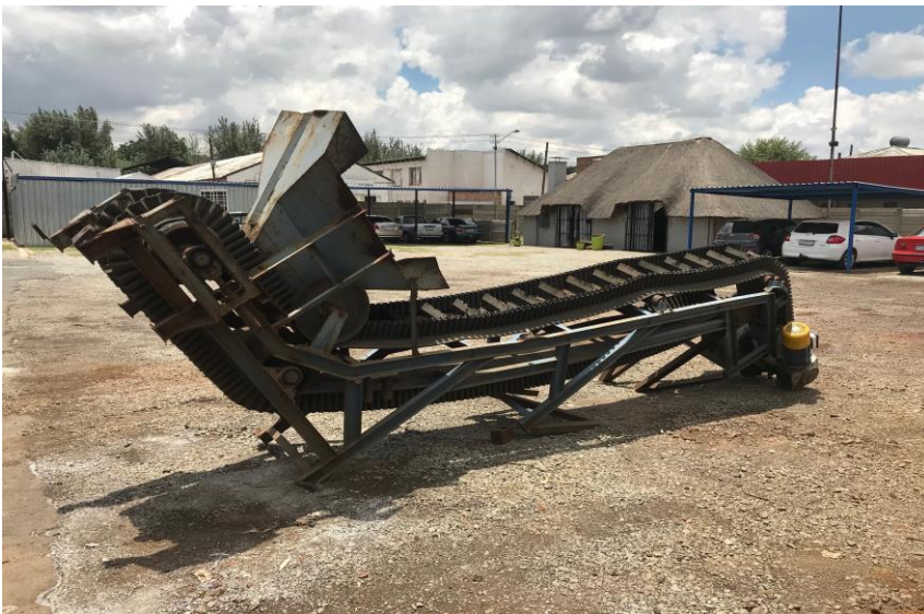
Image 3: Repairs to incline belt conveyor
